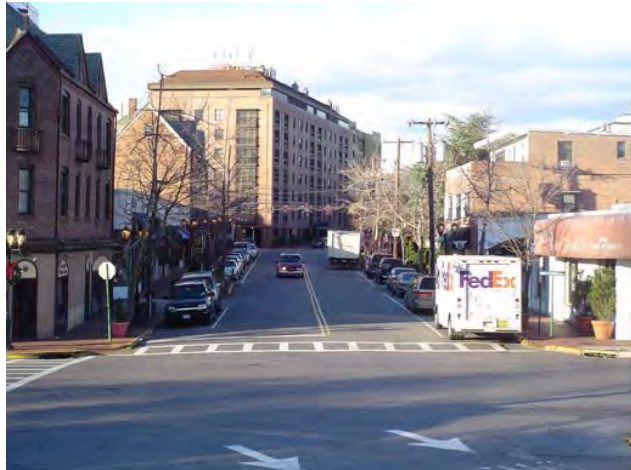
Figure 6 – Existing Bond Street conditions
