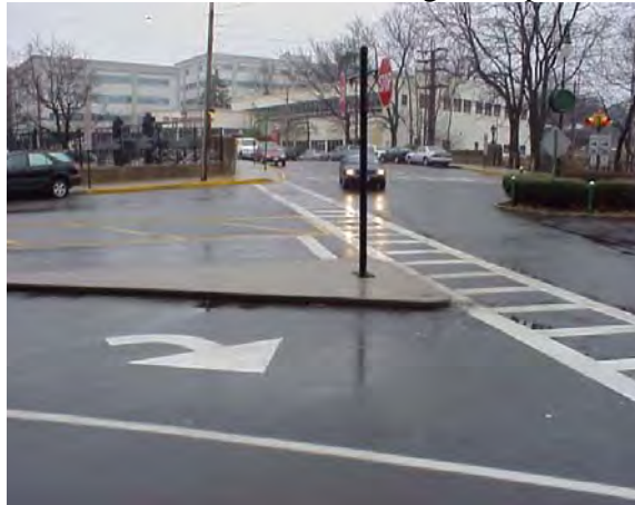
Figure 1 – “Before” construction of the roundabout at Barstow Road
