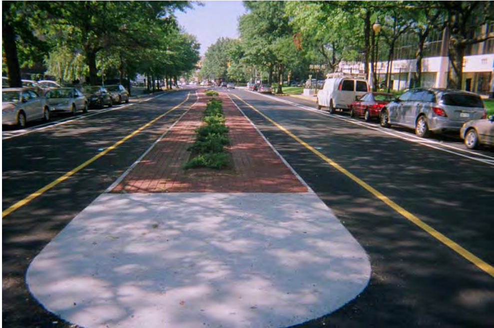
Figure 5 – “After” road diet construction on Great Neck Road
